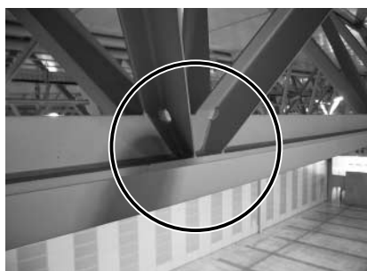
② Photographs of the ceiling frame for North Hall (Halls 9-11) and suspension plate
